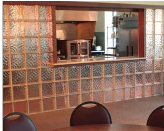
Glass blocks from the old Soup Kitchen incorporated into the Solanus Center Dining room.
